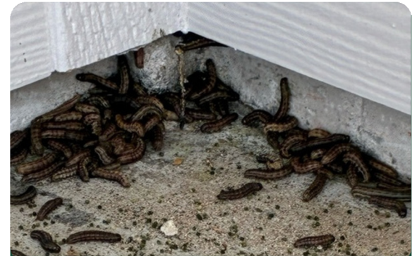
Armyworms along foundations
